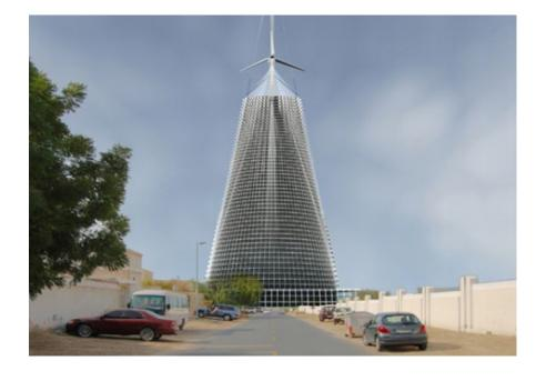
The 10 MW Tower (UNITED ARAB EMIRATES) is an eco skyscraper and renewable energy generating machine that harvests wind and solar power. A 5 MW wind turbine sits at the top of the building harnessing the wind, while the power of the sun is collected via a 3 MW concentrating solar system plus a 2 MW solar updraft system. Designed by UAE-based Studied Impact, this 50 story skyscraper will put out 10 times as much energy as it needs, pumping renewable power back into the Dubai electric grid.Â
