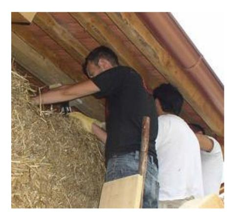
Straw-bale construction (USA/GB/IT) is a building method that uses bales of straw (commonly wheat, rice, rye and oats straw) as structural elements, building insulation, or both. This construction method is commonly used in natural building or "brown" construction projects. Advantages of straw-bale construction over conventional building systems include the renewable nature of straw, cost, easy availability, and high insulation value.
